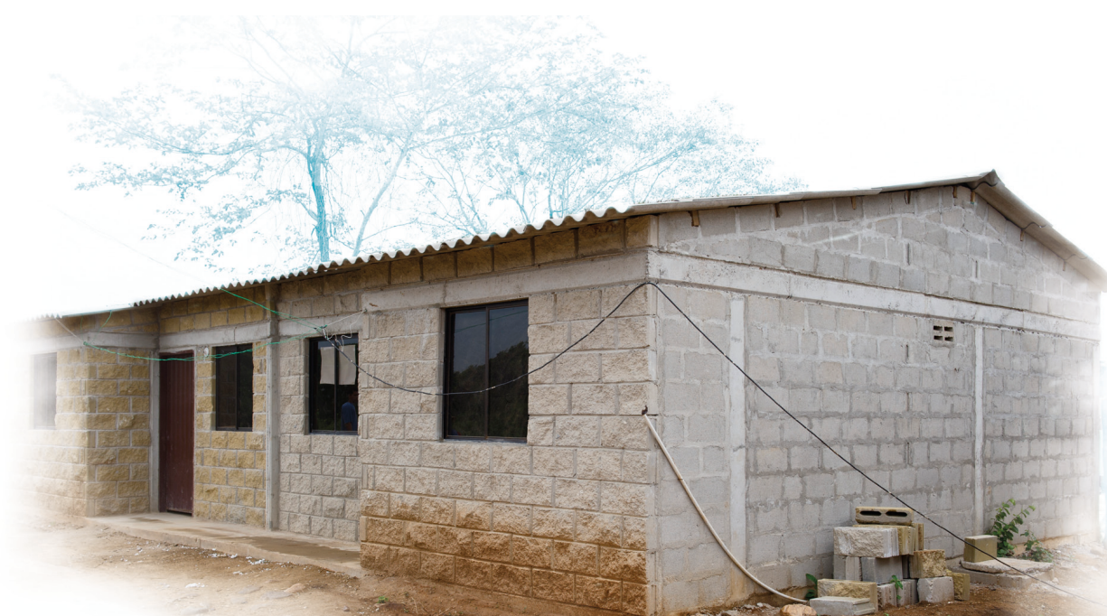
Houses built using Fair-trade banana premiums and company contributions. Located in Campana Nuevo, the houses are built and financed for the workers in the area.
