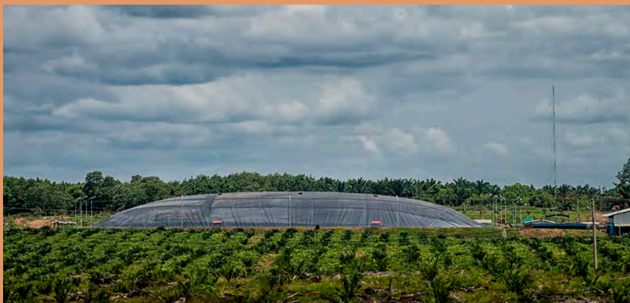
Methane Capture Facility
