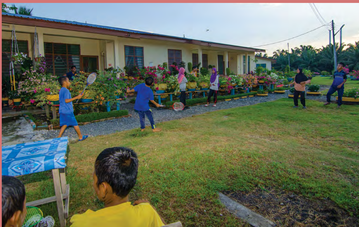
Plantation workers' housing complex
