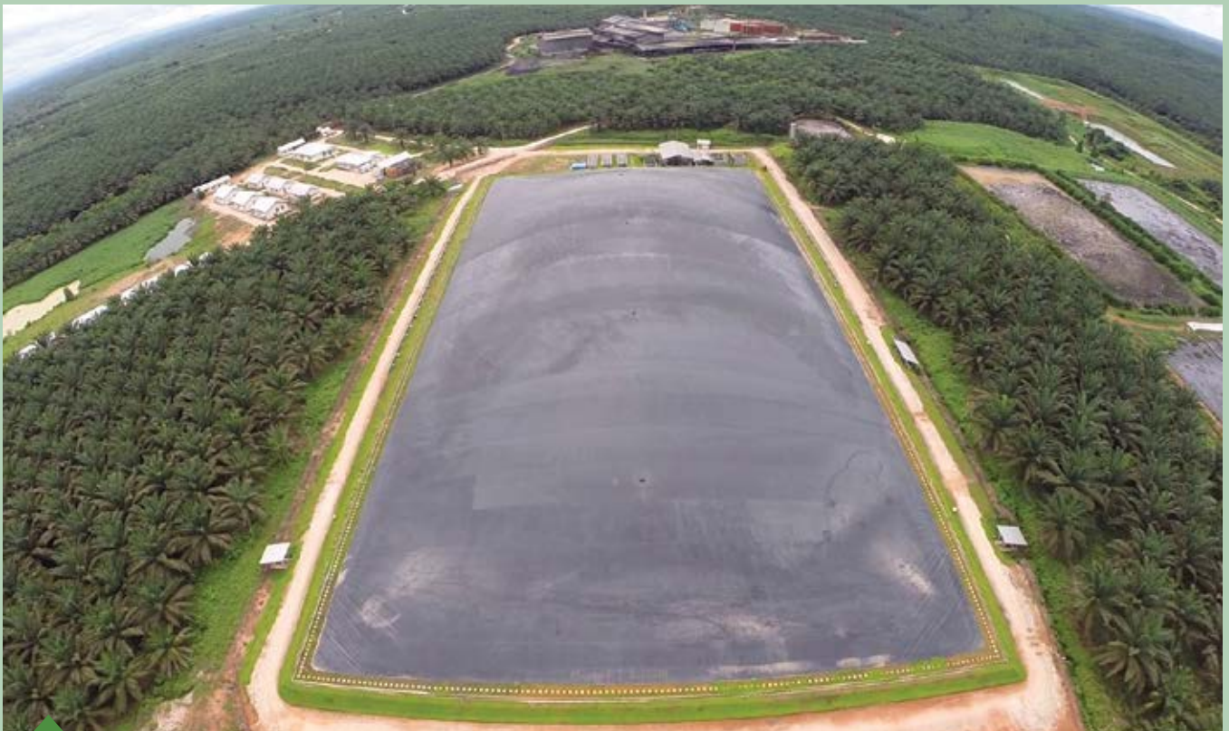
The methane capture plant at Cakra oil mill
