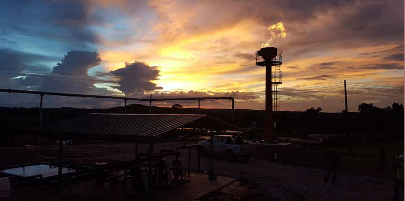
Flaring of biogas captured from the methane capture system in operation
