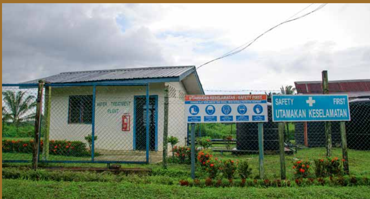
Safety boards with relevant warning signs are installed at areas with potential hazards
