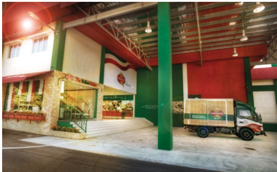
The Italian Baker's baking plant in Pulau Indah.
